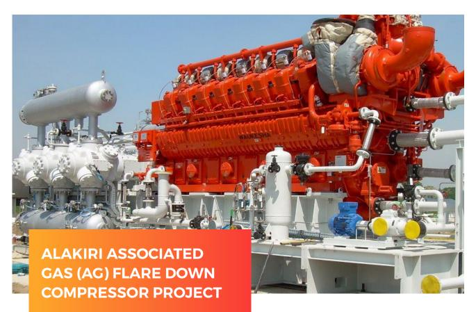
Client: Eroton Exploration and Production Company Location: OML 18, Alakiri Field, Rivers State. Scope: Installation and Management of two Associated Gas (AG) Compressors Capacity/Flow Rate: 7MMscf/day each Start Date: January 2021 Status: Ongoing
